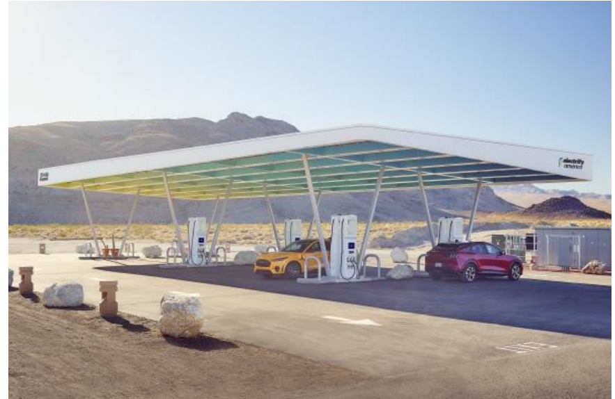
Electrify America EV fast charging station with solar-powered canopy located in Baker, CA. Image credit: Electrify America
