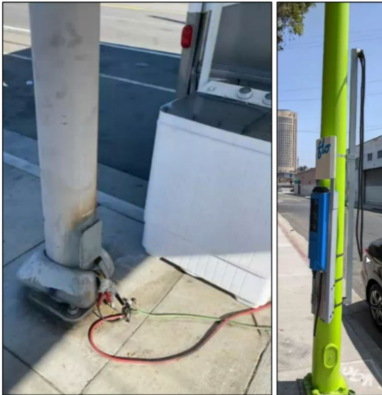
Examples of charger vandalism challenges. Power is redirected to a washing machine (left). A cut charging cable (right). Source: City of Los Angeles
